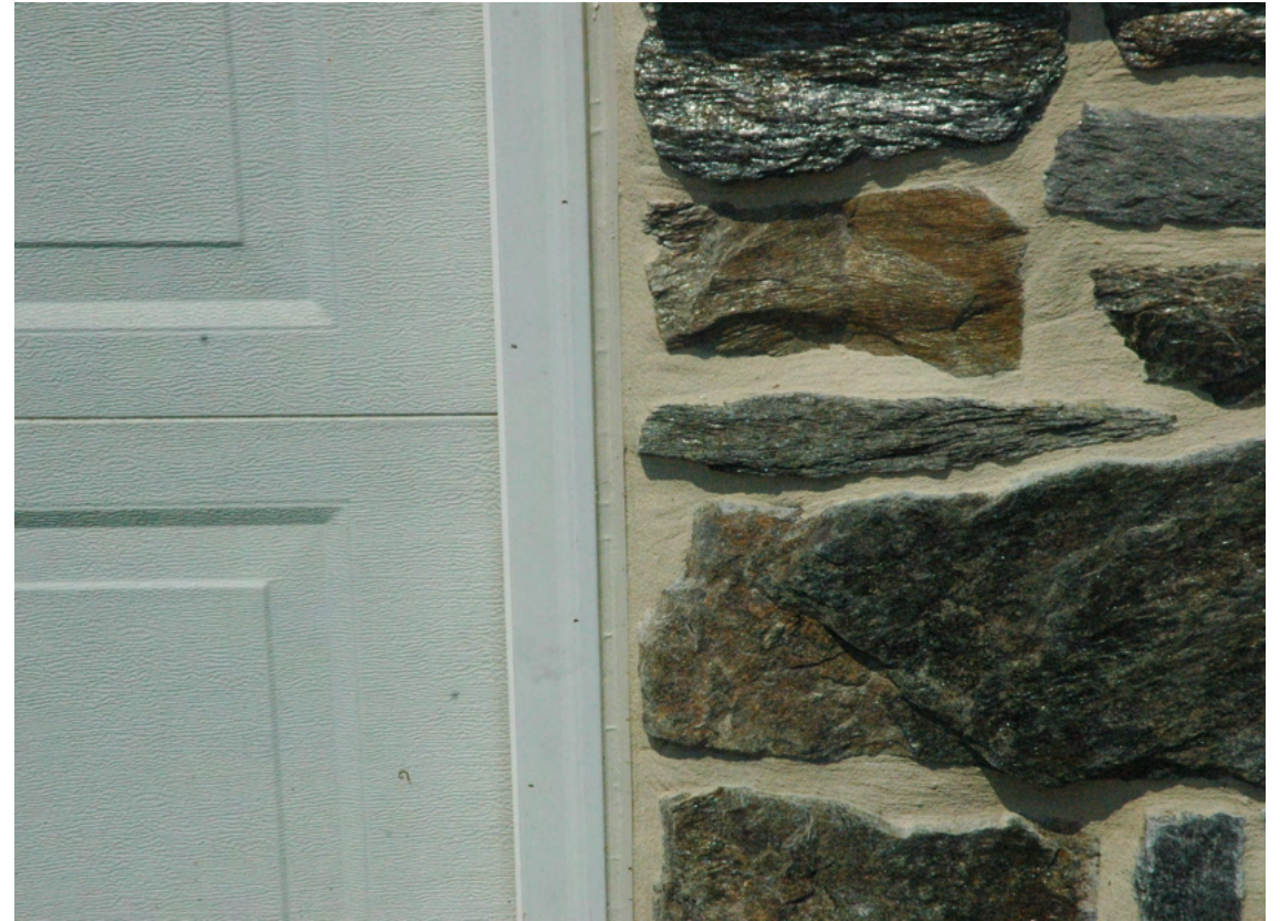
Code Compliant – Note Caulk Joint
